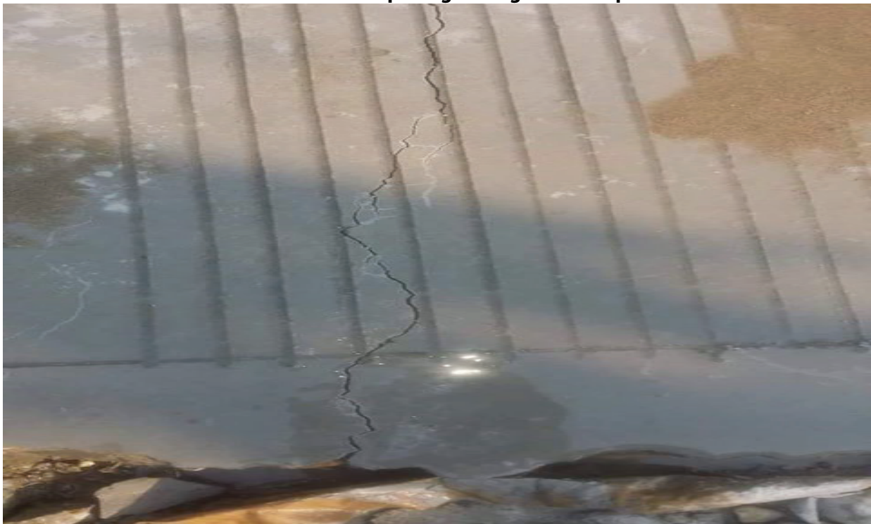
Picture1. Road Built Before the Official Opening in Hlegu Township
