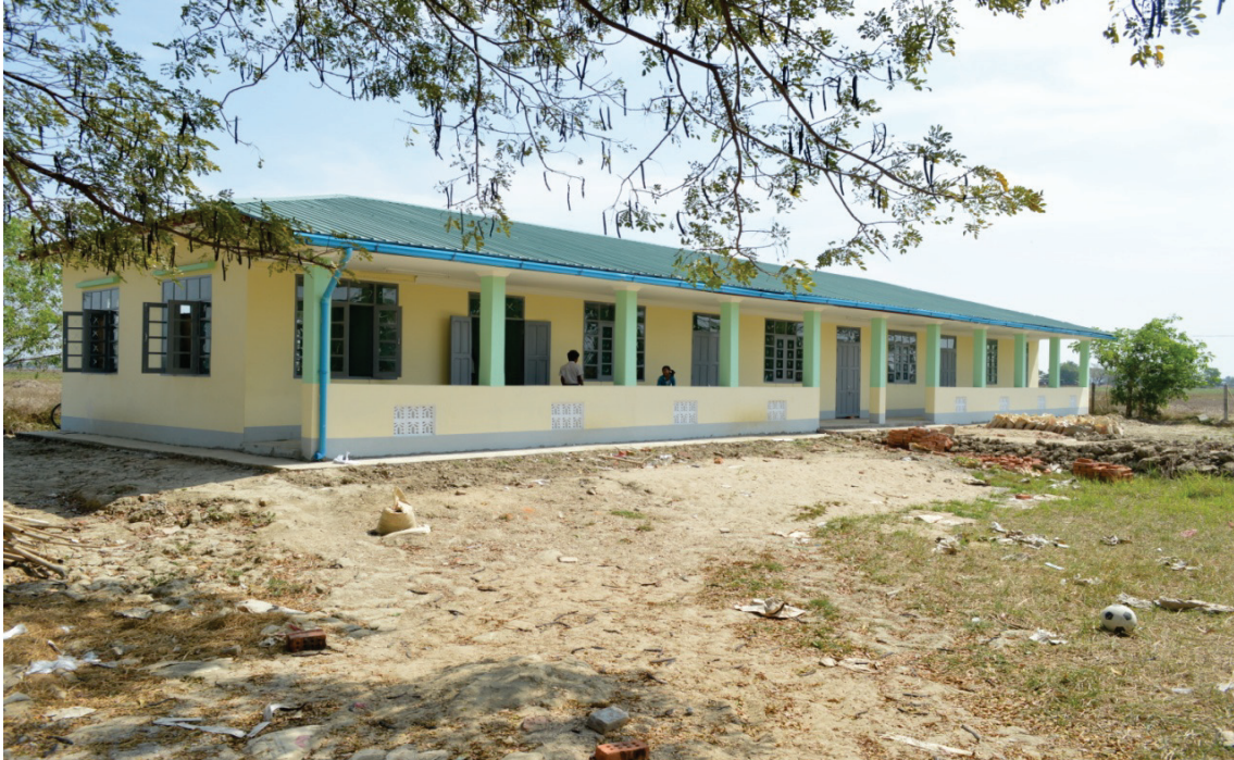
Picture 4. Basic Education Middle School ( Kan Pa ) (90% completed)
